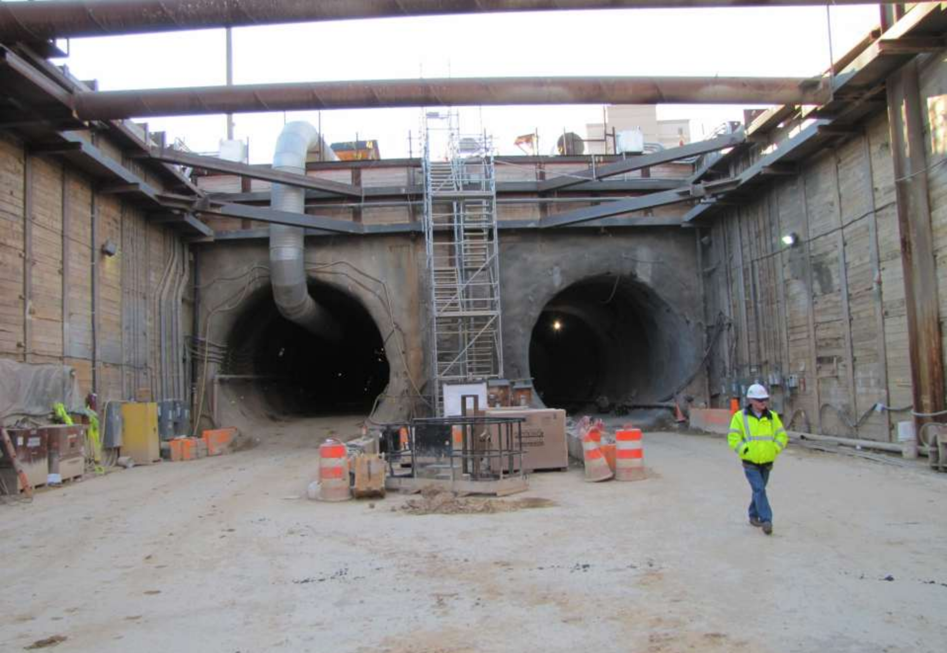
Inbound & Outbound Tunnels complete
