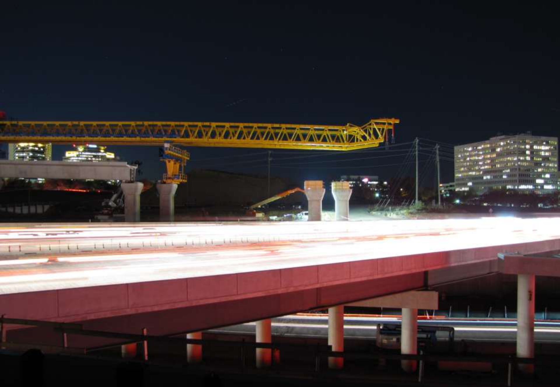
Truss overlooking the Capital Beltway
