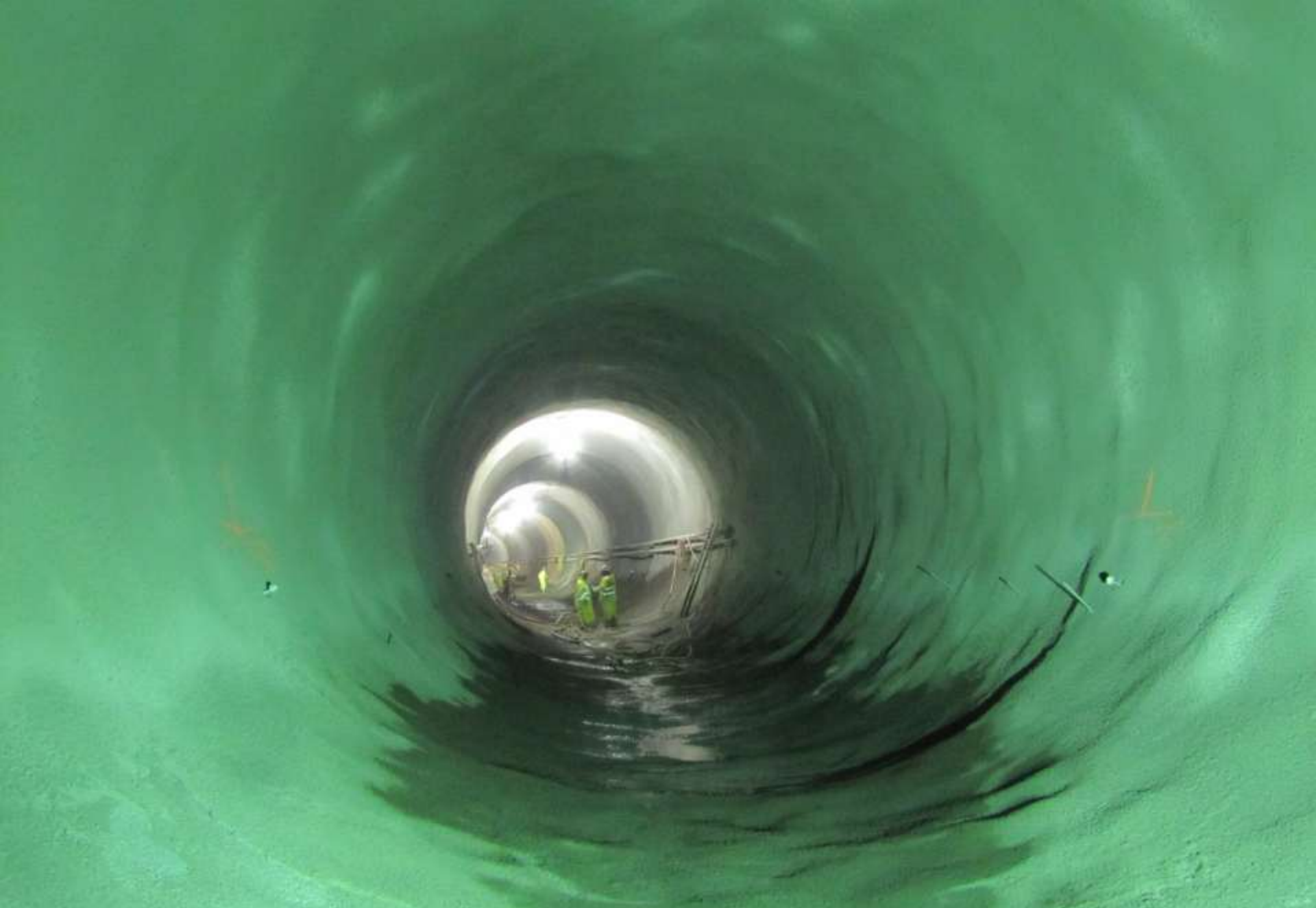
Interior of Tunnels covered in shotcrete
