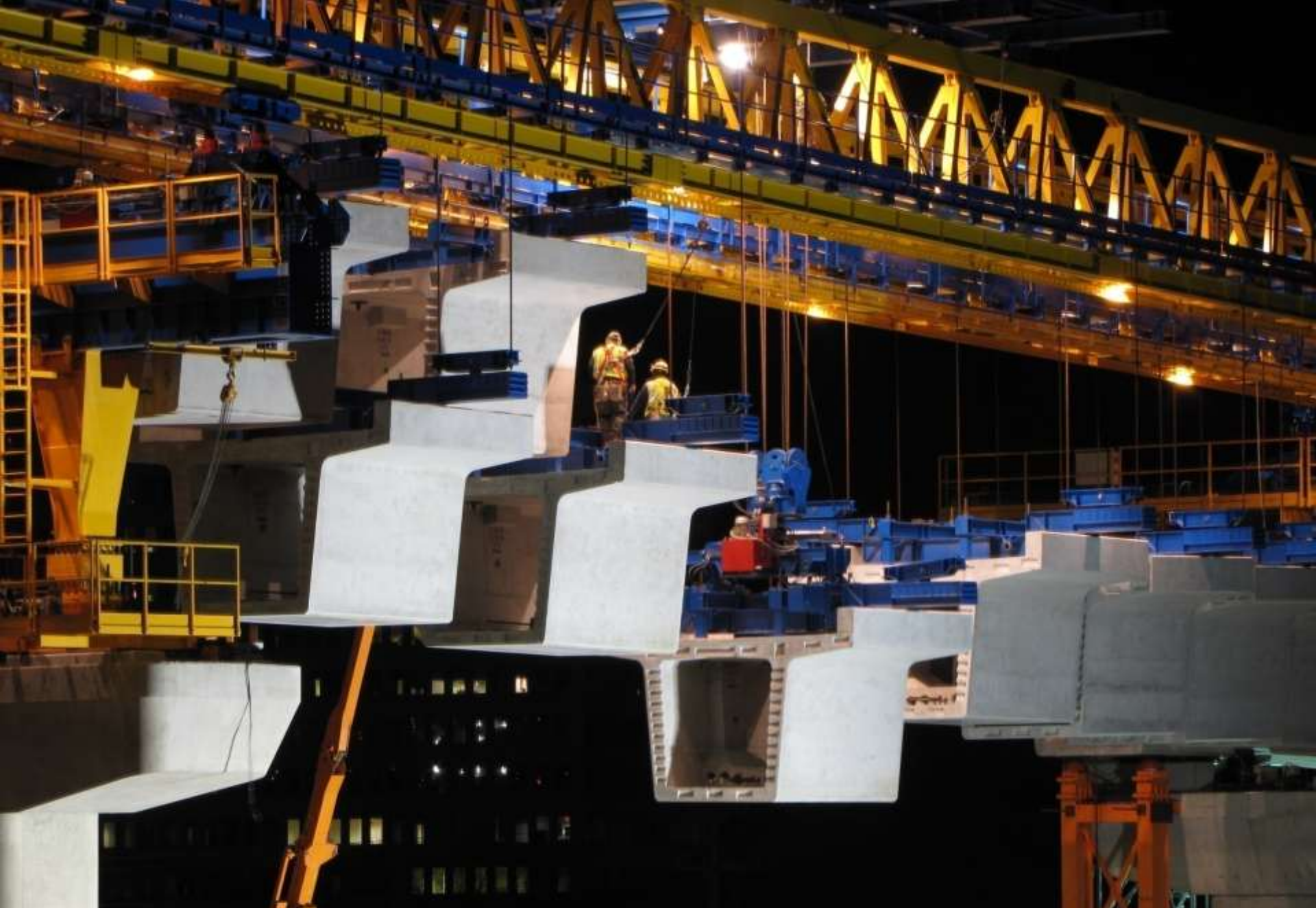
Concrete segments being erected for spans
