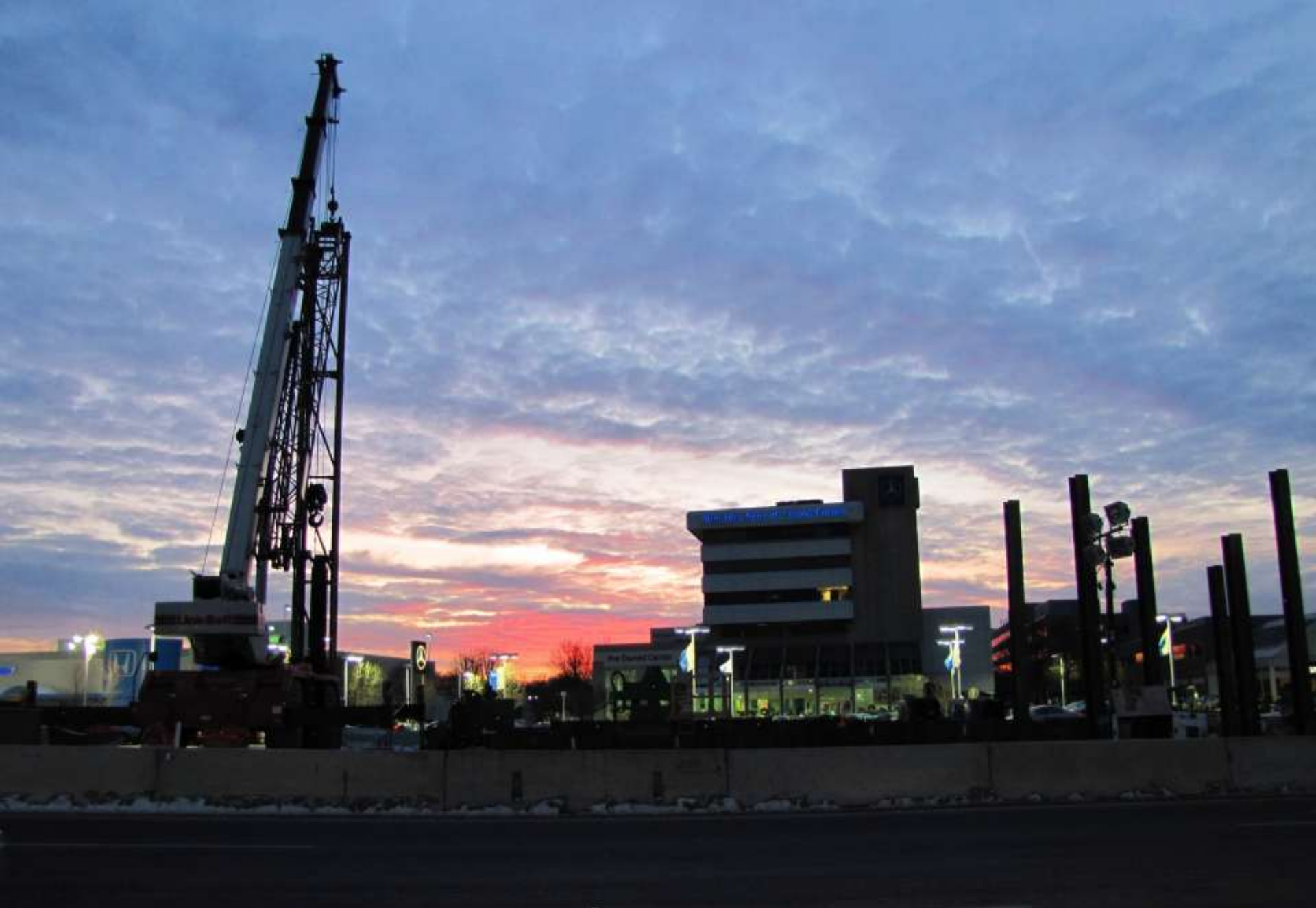
Tysons West Station Construction
